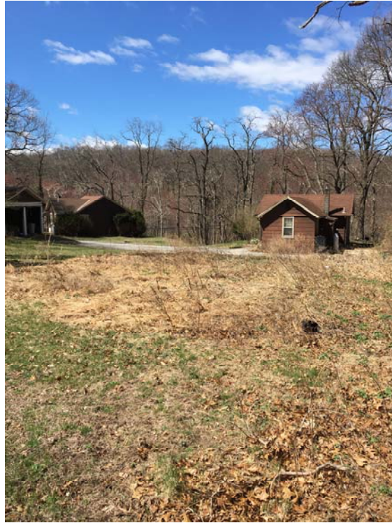
31: View looking west within tax parcel 3.3, towards existing structures proposed for removal, near Lee's Court western entrance from Makamah Road.
