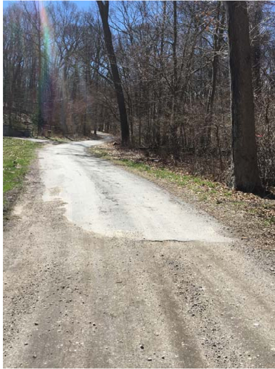
29: View of private right-of-way off Makamah Rd., looking south towards east entrance of proposed Lee's Court.
