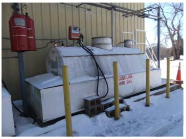
View of above ground diesel storage tank for equipment shed
