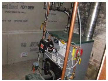
View of fuel oil-fired boiler in basement of pro shop
