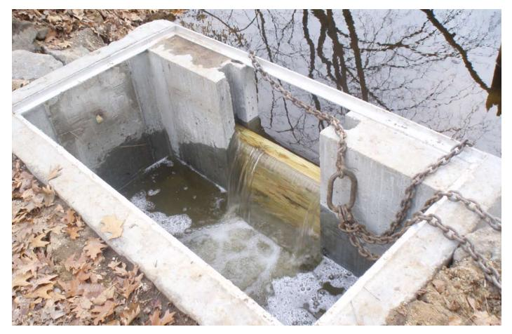
After placing the adjustable wooding barriers, Fuch's Pond begins to return to it's 'original' level.
