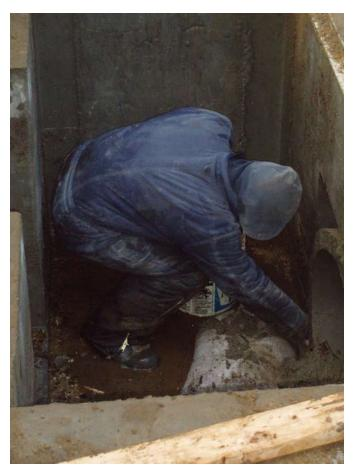
Sealing the connection from the inside of the outflow box.
