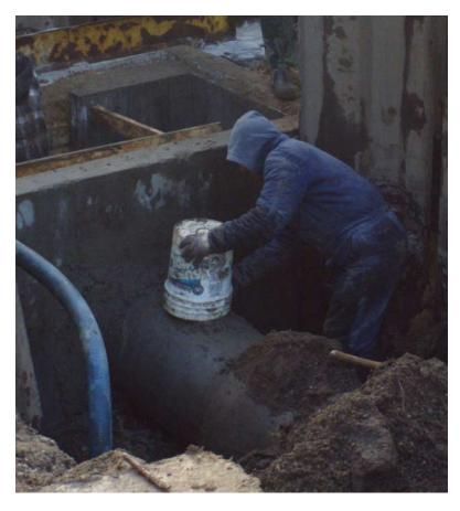
Sealing the connection from the ourside of the outflow box.
