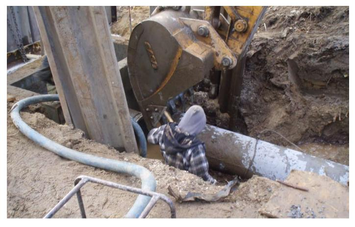
Connecting the new outflow box to the pipe.
