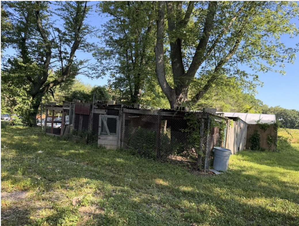
Photo 3 – View facing northwest towards old coop structure on Project Site.
