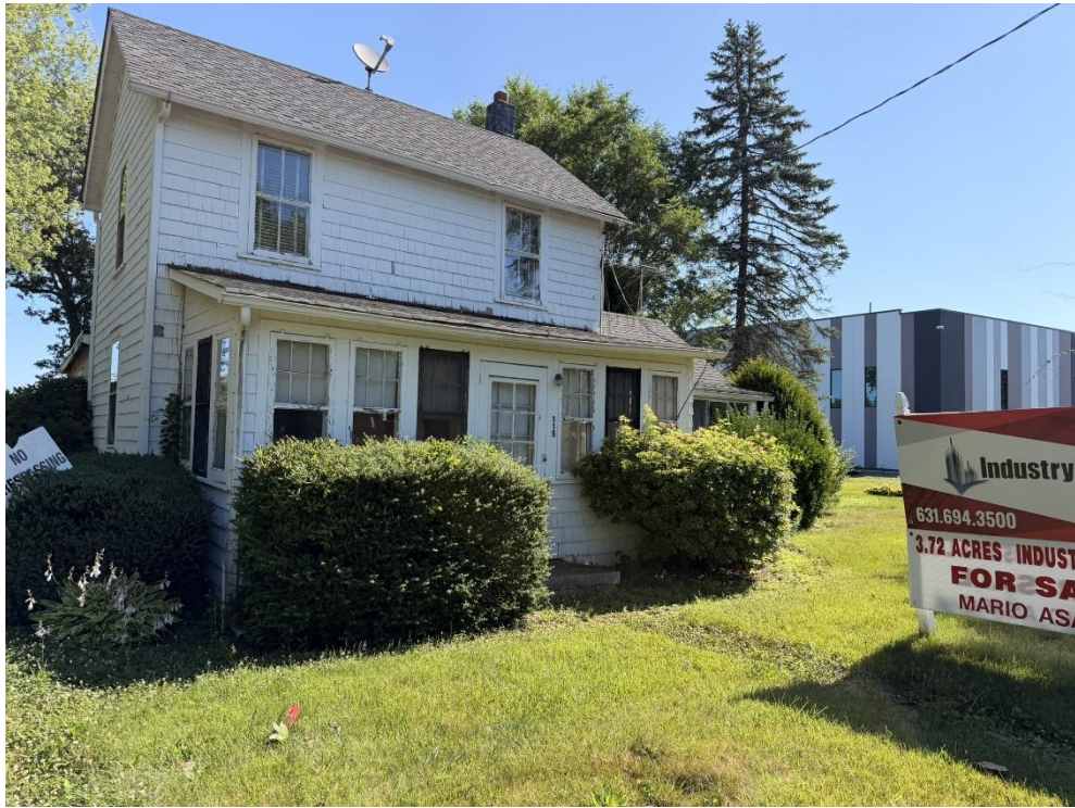
Photo 1 – View facing northeast towards vacant residential structure with commercial facility in the background.
