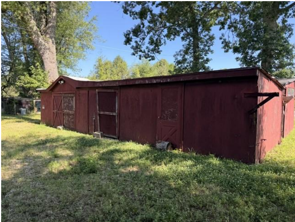
Photo 4 – View facing north towards old agricultural structure on Project Site.
